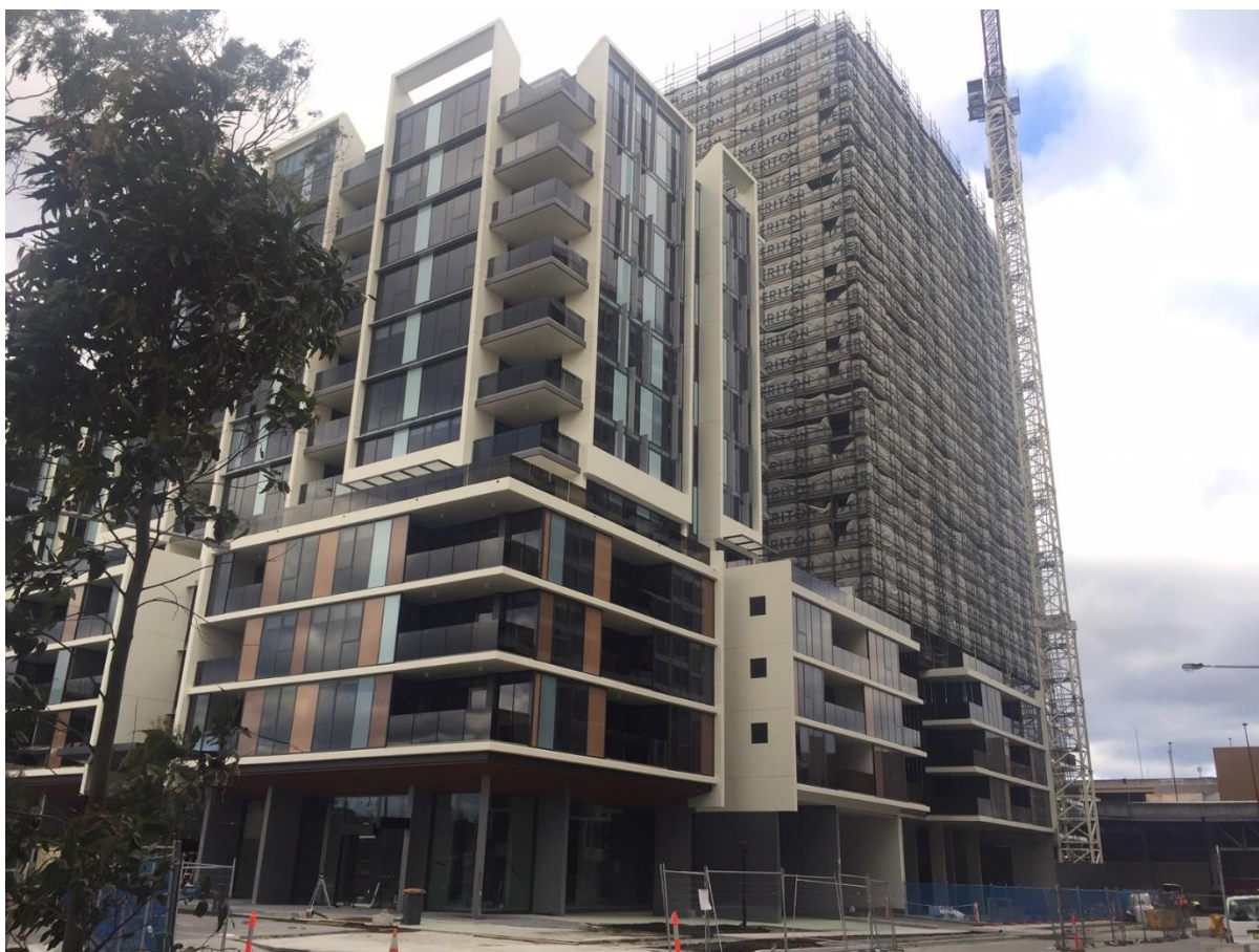
Figure 3 UB5C currently under construction. Note the porte cochere area has been left hollow.
